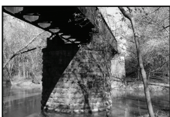
Hand-cut stone of original 1884 bridge. Photo by Tom Woodward.
