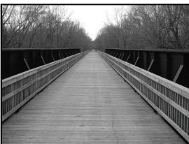
The current auto lane ready for traffic!
